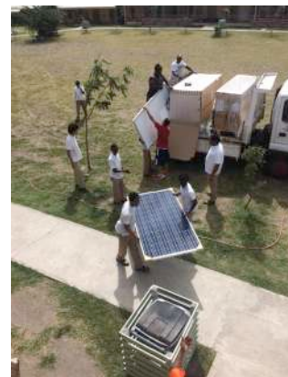
Pupils at the St. Anthony's Secondary School unload panels for their 14KWH system
